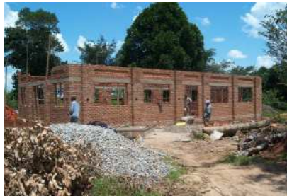
Walls going up on
