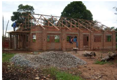
Roof going Front & Side View
