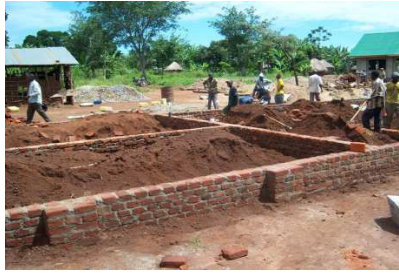
Foundation for New Side View of School
